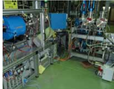
The MedAustron low-energy test beam line at CERN: from the particle source (blue cylinder) the beam passes through a spectrometer dipole (blue, in the centre). Vacuum tanks with beam diagnostics for analysing the particle beam are installed on the right.
